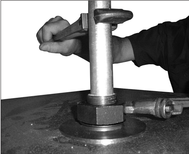
7b. Verify that full contact has occurred between the sprinkler plate and freezer ceiling, as shown above.
