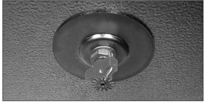
7b. Verify that full contact has occurred between the sprinkler plate and freezer ceiling, as shown above.
